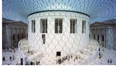
Figure 3. English Museum glass roof extension (Kayan, 2020).
