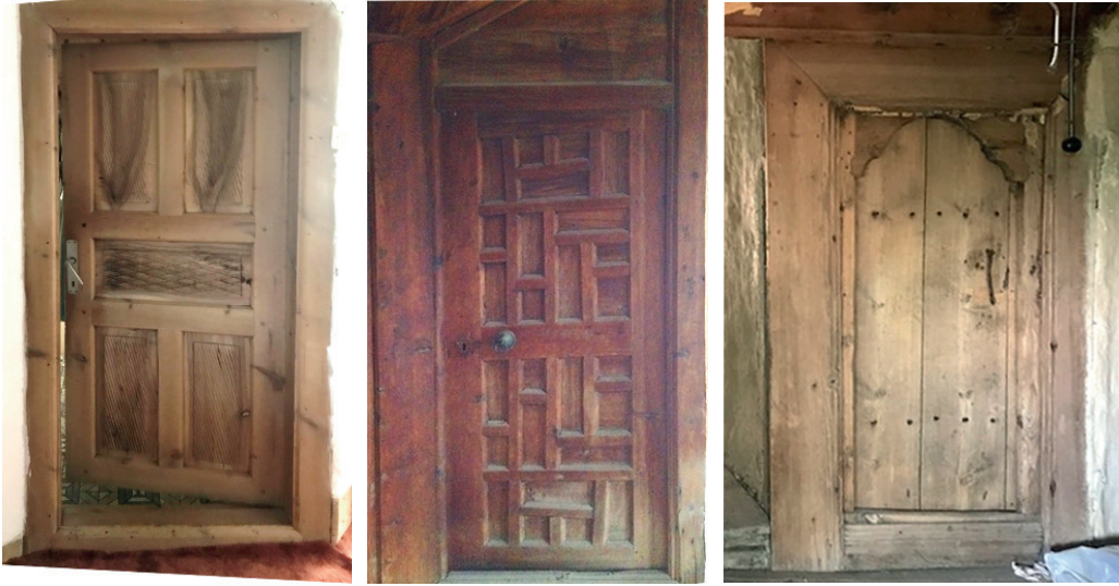
Fig. 12. (a) 5-panel door; (b) the door is decorated with various geometric shapes; (c) the door with a hood
