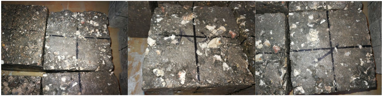
Fig. 15 Freezing and thawing damages for RCC specimens after 300 cycles
