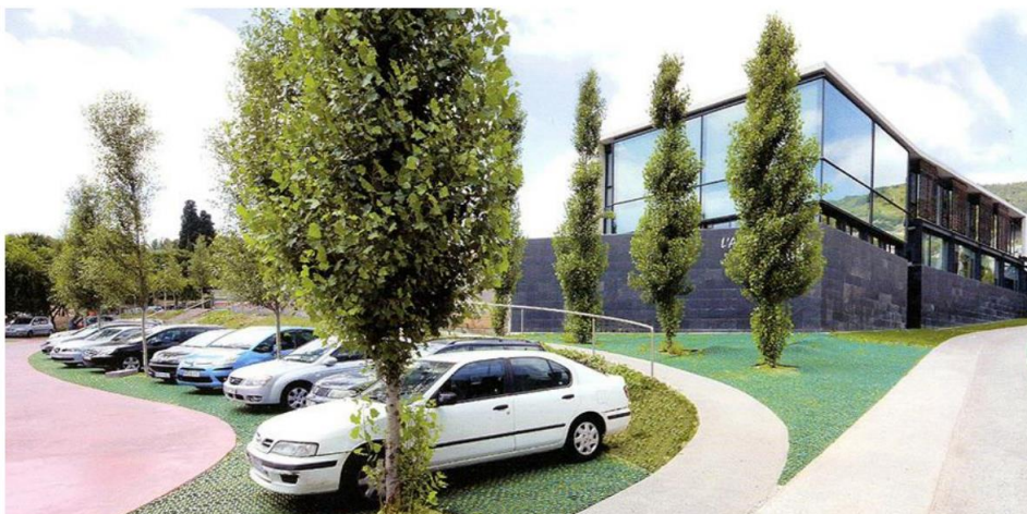
Figure 16. Figure 3.10 - Detail of Can Caralleu Parking lot and street. Different pavements were used. Almost half of the total area of intervention includes permeable pavement. Source: (Vidiella & Zamora 2011, p.160; Silva & Costa, 2016)
