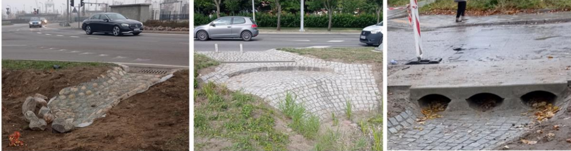
Figure 8. Examples of existing entrances from rain gardens in Gdańsk (photo by M. Kasprzyk)
