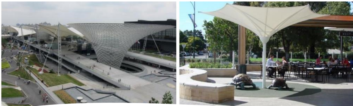
Figure 19. Left: Mega water collection structure on Expo Shanghai boulevard. Image credit: Tonylaw, 2010. Right: Inverted umbrella implemented in a small playground at the Woolworths Shopping Centre in Walkerville, Australia. Image credit: Universal Magazines Pty Ltd, 2013)
