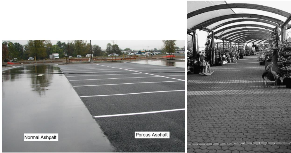
Figure 15. Porous asphalt. Porous asphalt (Silva & Costa, 2016)
