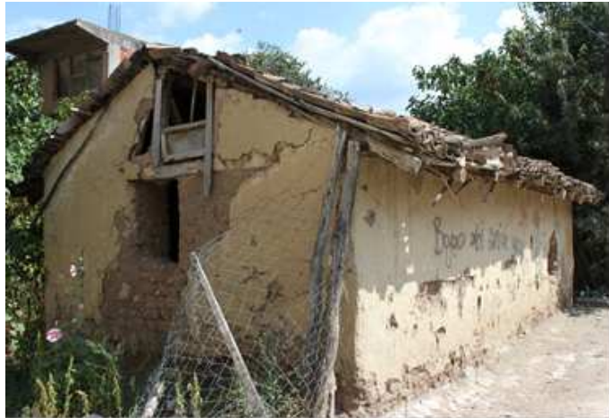
Figure 5. A barn with load bearing system
