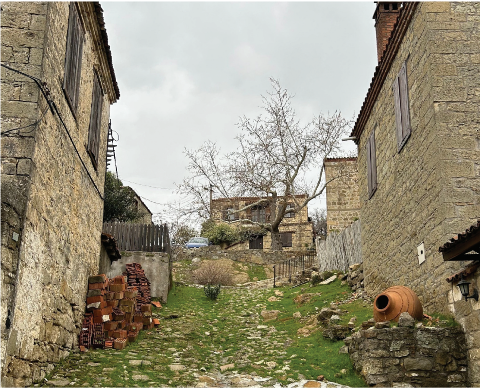
Figure 4. The historical buildings in the village, with their stone architecture.
