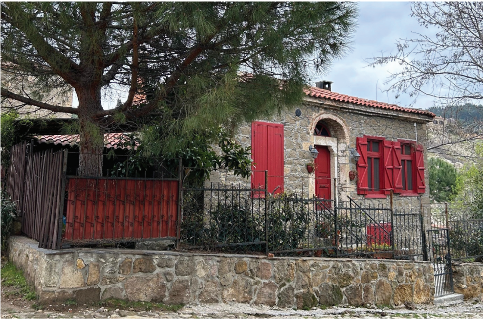
Figure 3. Restored old stone house.
